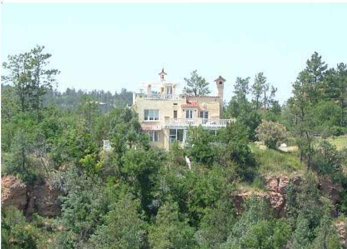
Hazardous fuel loads on the slope below this structure put it at risk from the possibility of extreme fire behavior.
